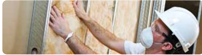
CertaPro™ Commercial Insulation
